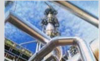
Process Control Systems
